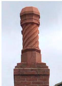
Existing chimney pot
